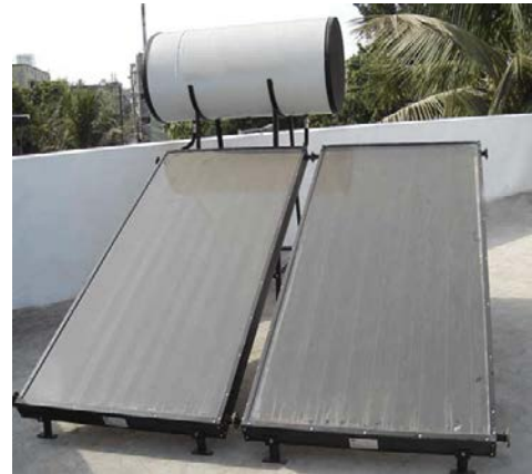
Figure 2: Solar water heating system
